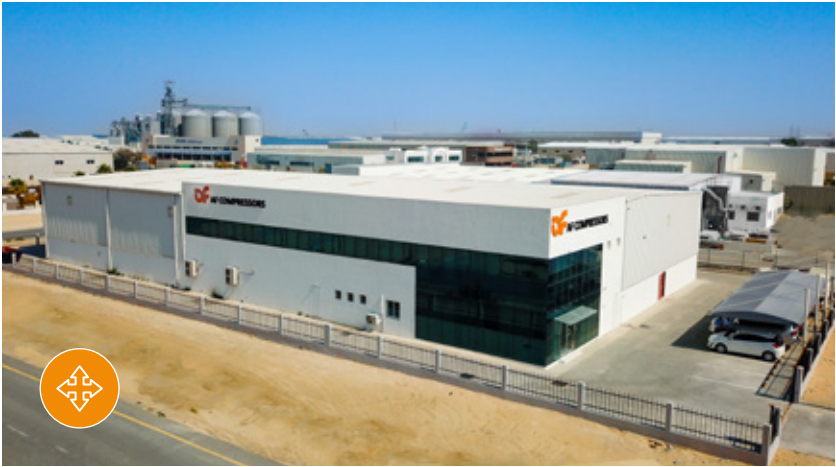
AF MIDDLE EAST FZE IN UAE DUBAI Distribution center
